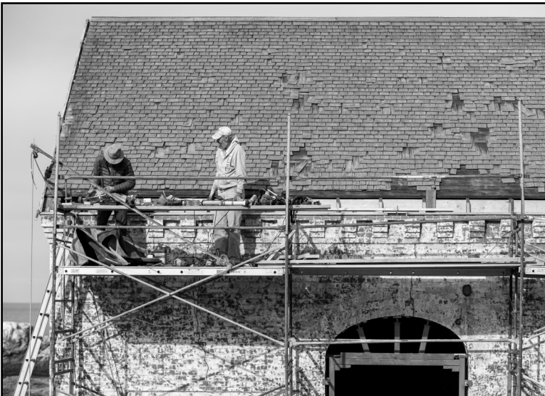
Before: The roof leaked and had missing shingles.
