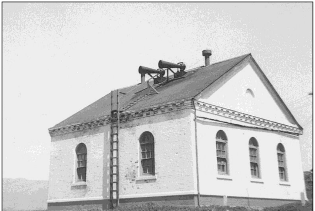
Fog signal building circa 1938, with Type G diaphone signal (below).
