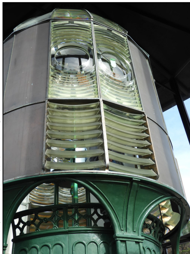
Above: The upper glass prisms and bullseye panels shine after their initial cleaning. Note the bottom two panels are dull with years of grime.
