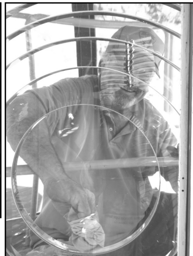
Above: There was room for a 6 foot ladder inside the lens! Right: After polishing, the bullseye panels were clear enough to see through again.
